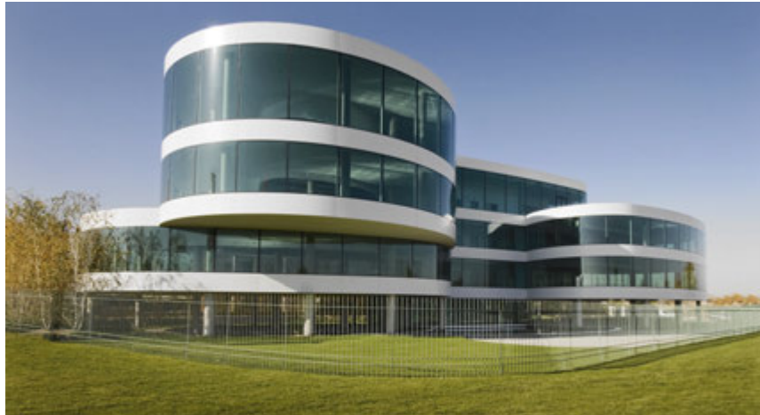
New Corporate Offices in Madrid (Spain)
